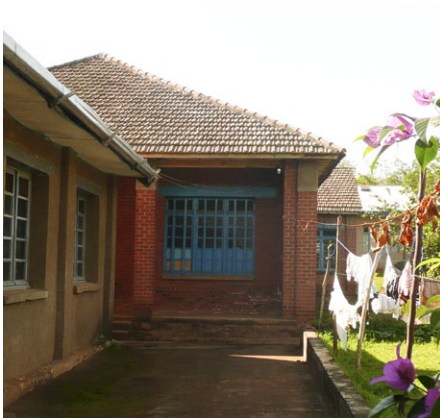
1. The outside path of the orphanage
