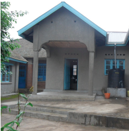
3. The new building comprising a kitchen, a dining area and a playing area
